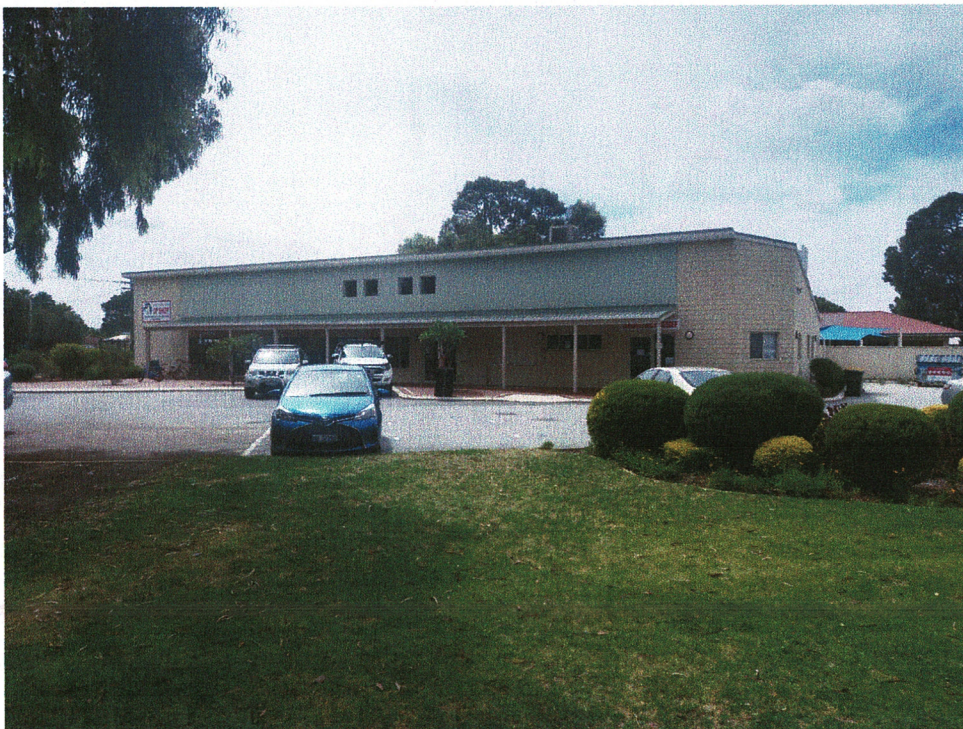
Church of the Way 'Rafters' complex which is adjacent to the worship centre, consisting of an Op Shop, Offices, Commercial Kitchen, large Dining Room, Emergency Relief, showering facilities and toilets.
